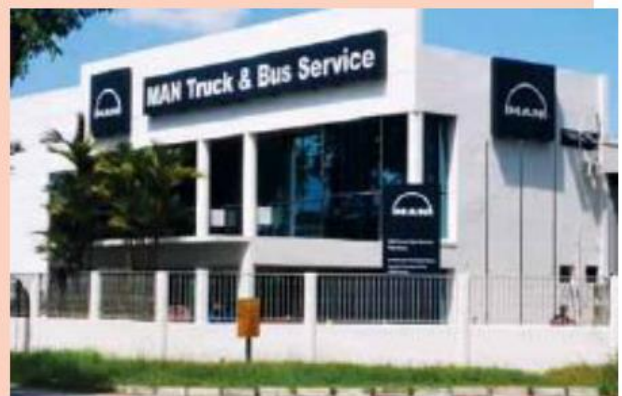
Prai Service Centre
