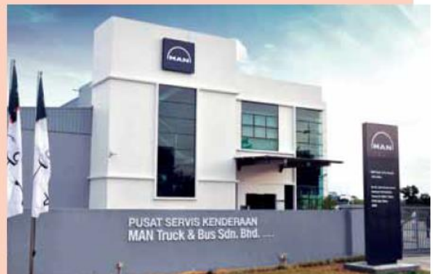
Johor Service Centre
